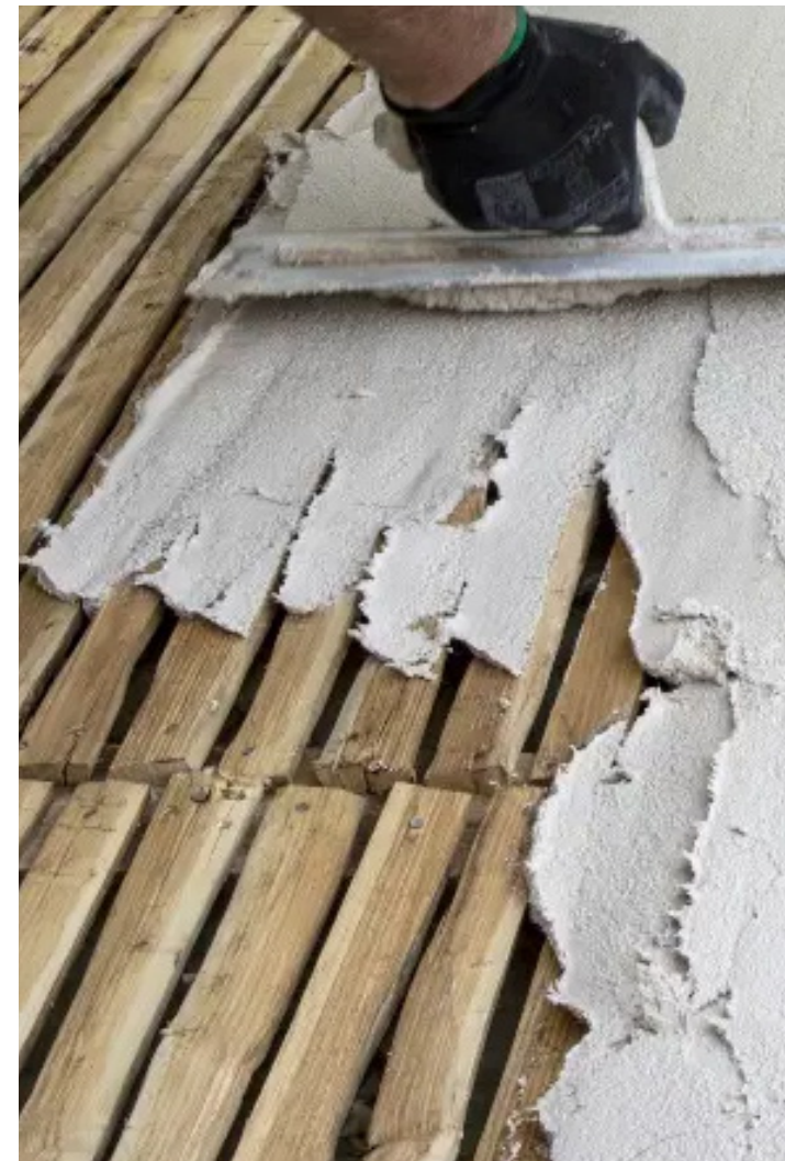
The lime and lath technique
