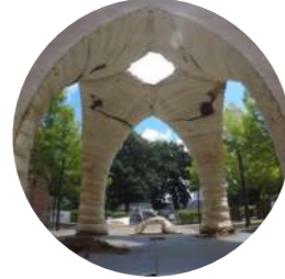
Monolito Micelio, MycoMatters Lab, 2018 Wooden internal reinforcing; mycelium processed on-site, packed into the plywood and geo-textile formwork;
