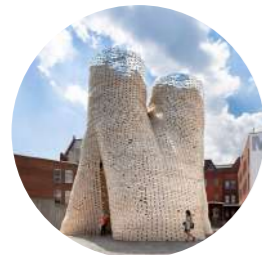
The Hy-fi Tower, The Living, 2014 12 m tall pavilion that used 10,000 mycelium bricks
