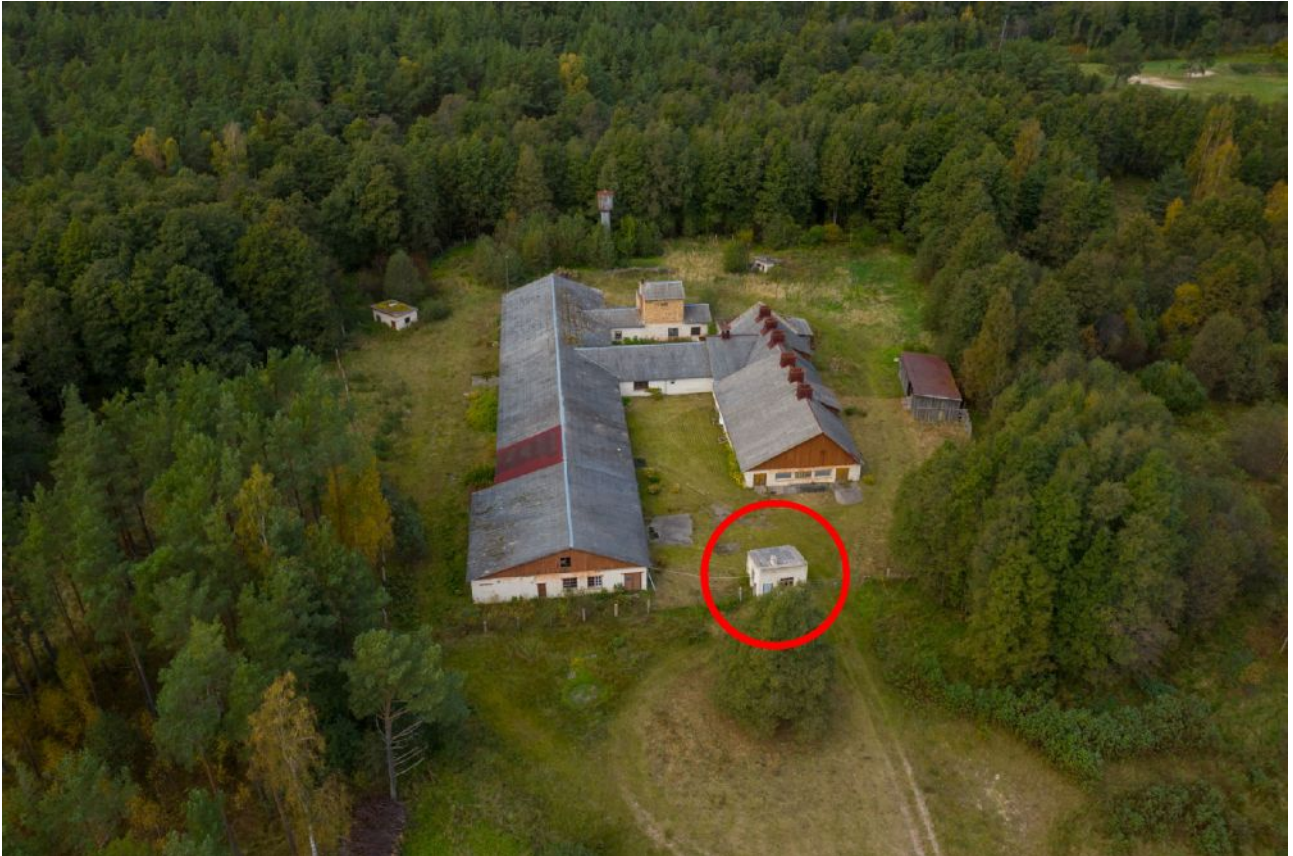
Pitrags Pavilion before refurbishment / areal view
