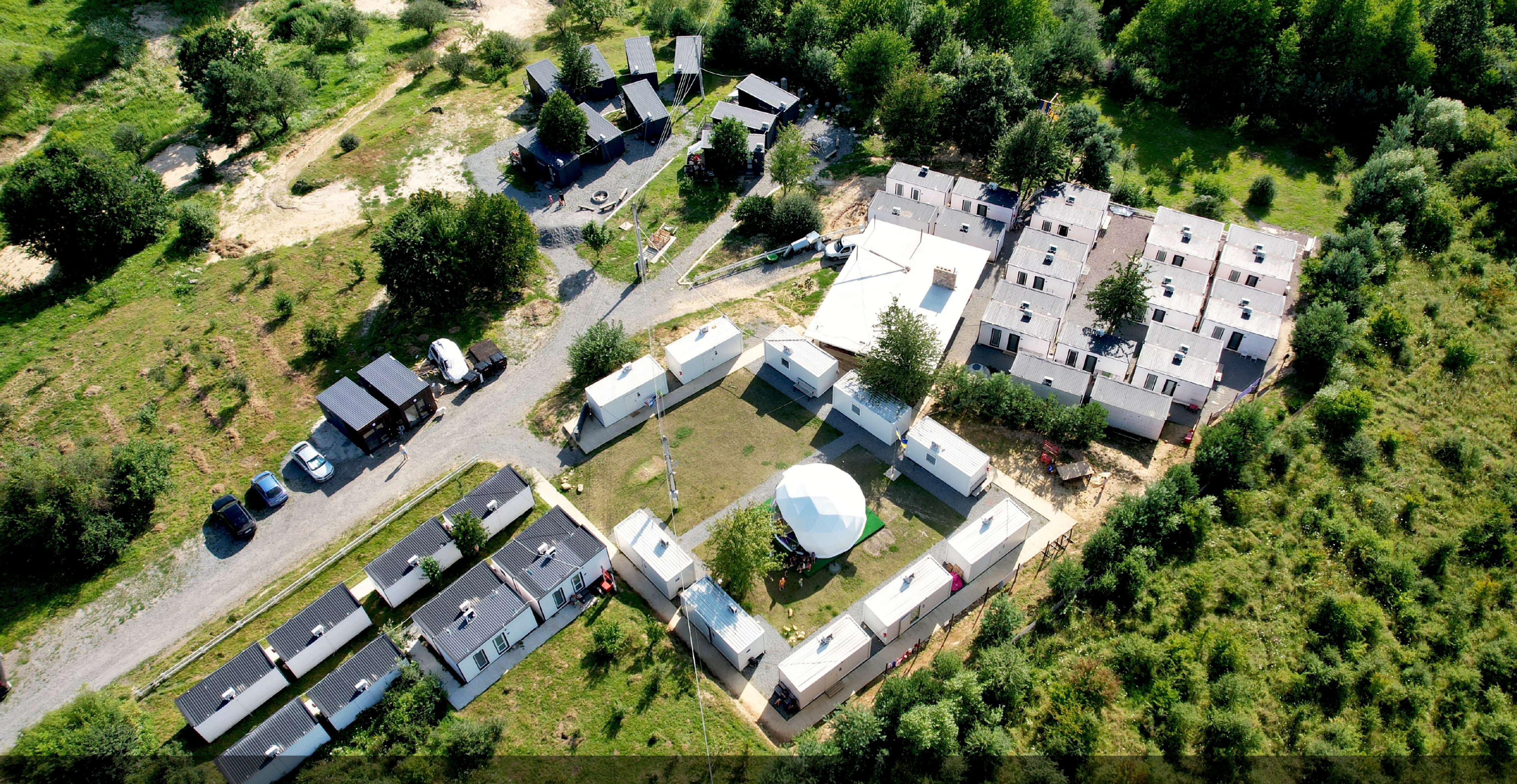
LARGEST PRIVATE MODULAR SHELTER IN UKRAINE FOUNDED IN APRIL 2022
